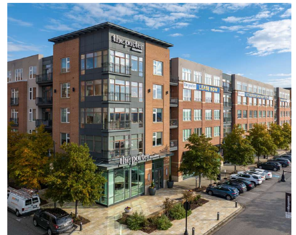
High-rise Apartment Buildings
